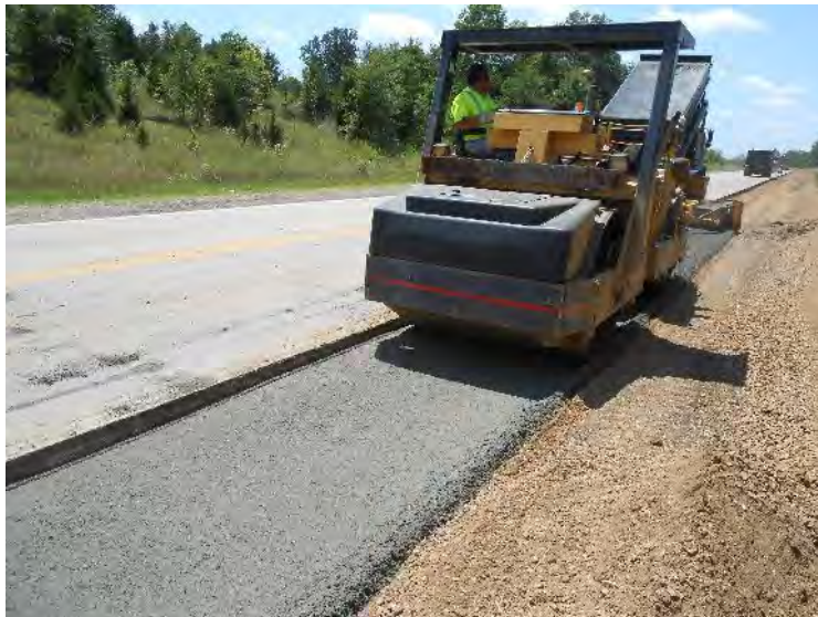
Figure 34: Compaction of RCC above installed sensors
