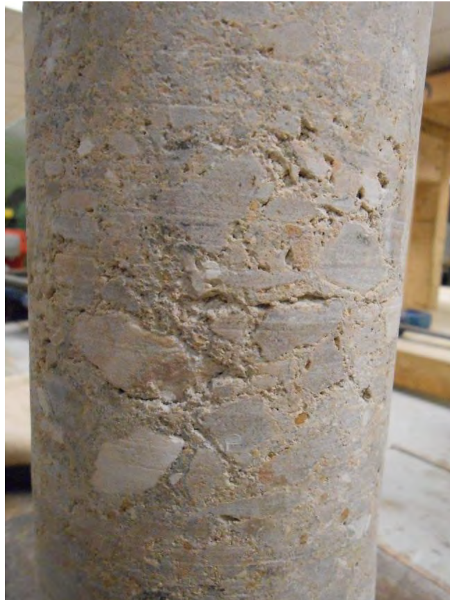
Figure 25: Joint between two casting layers showing increased porosity as observed for core C2
