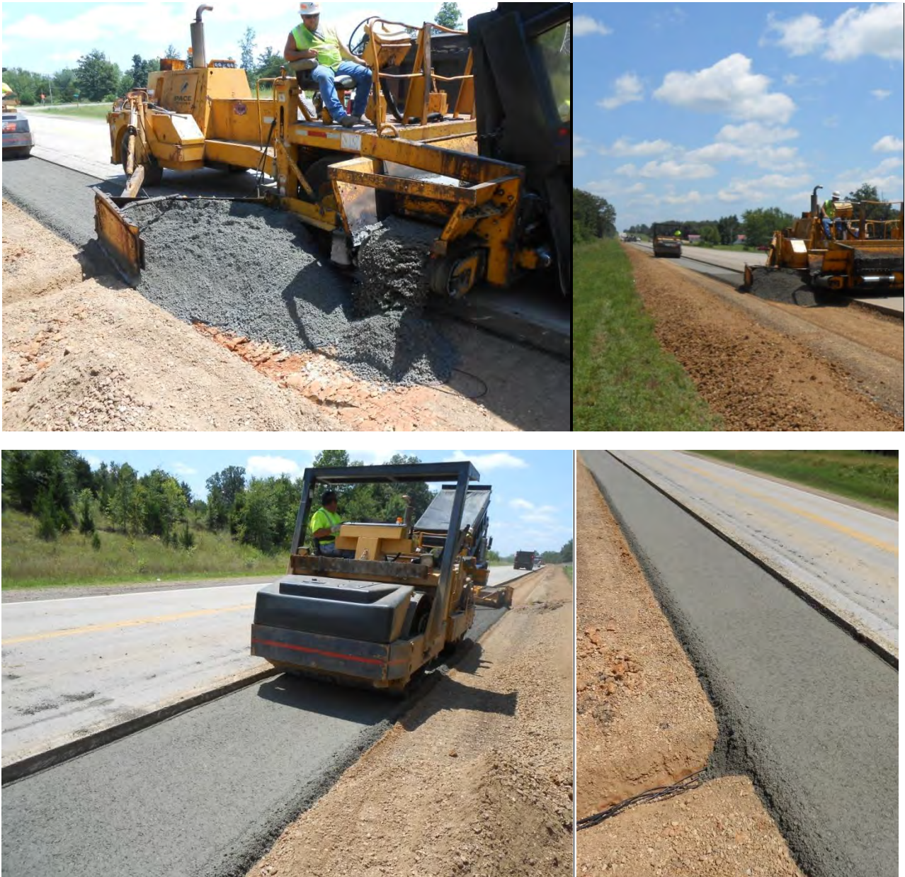
Figure 19- RCC pavement construction in Route 160
