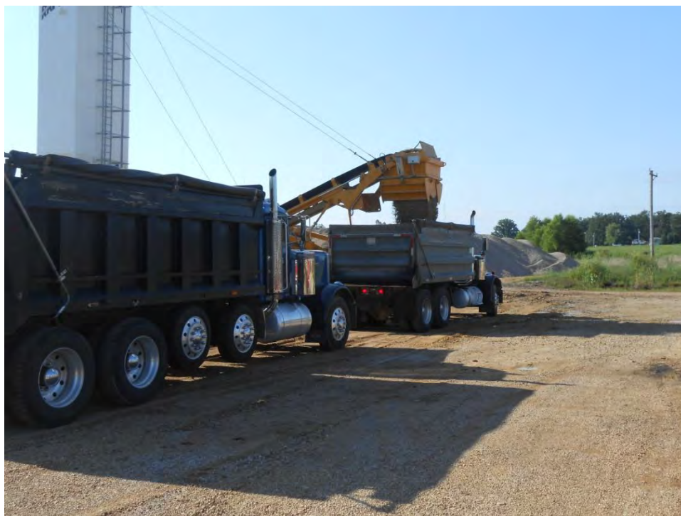
Figure 18- RCC production facilities used for widening Route 160
